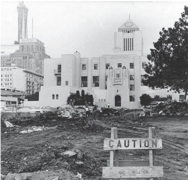
The original Central Library gardens are shown being demolished to make way for a staff parking lot, 1970. (Herald Examiner Collection)
