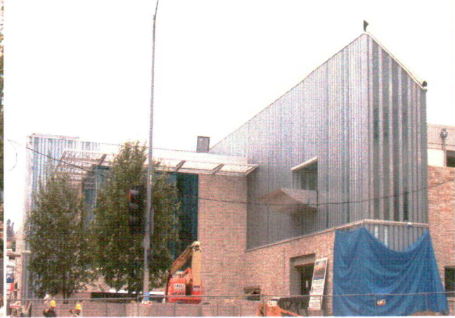
Plaza Area/Main Entrance
